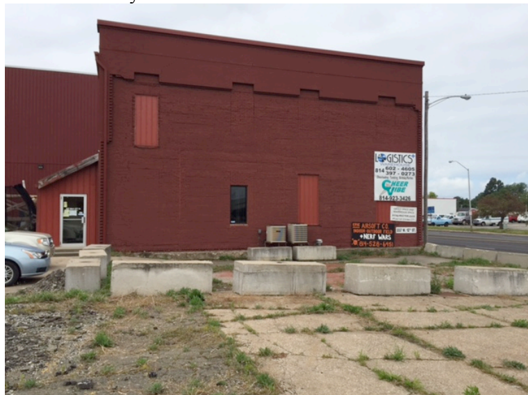
The wall is approximately 50 feet wide and 30 feet tall.
